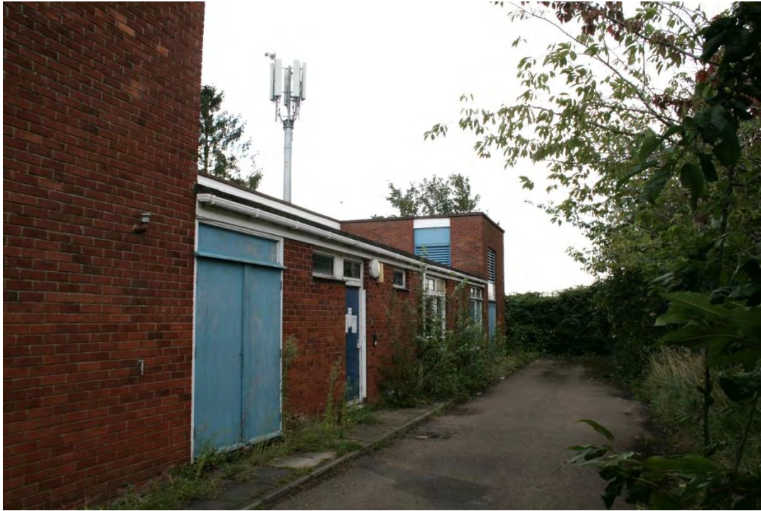
5.6 Telephone Exchange and Phone mast on East side of Weeping Willow
