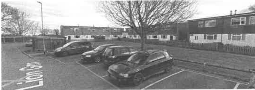
Fig. 6 – view of buildings & electrical sub-station near Barrow House
