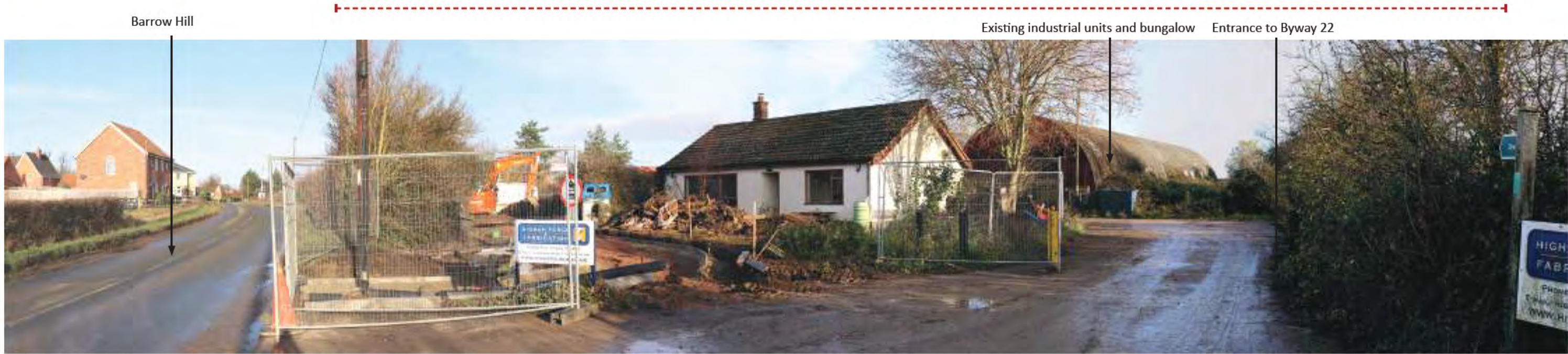
View 9: Looking north along Barrow Hill with proposed site to the east with existing industrial area and Hopkins development obscured
